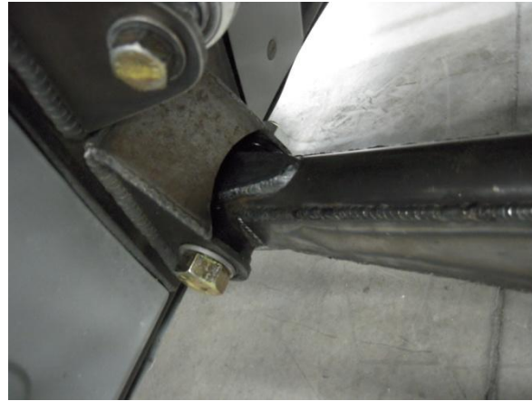
Top View of installed wrap on lower trailing arm
